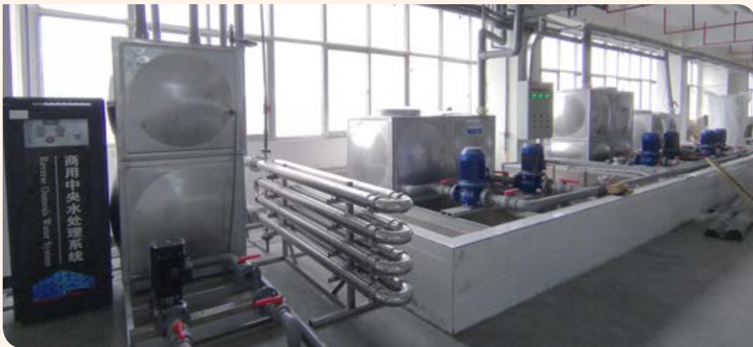
Water Circulation System in Xiamen Plant 廈門廠房的水循環系統
